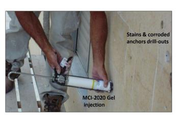
MCI®-2020 Gel has been proven to be a successful alternative to topical treatments. One example of use is the repair of stone clad residential buildings in Israel. These buildings had an architectural style consistent with others in the region, which is known to have problems with corrosion of both reinforcement and stone cladding tile anchors, causing tiles to detach and start falling off a relatively short time after
